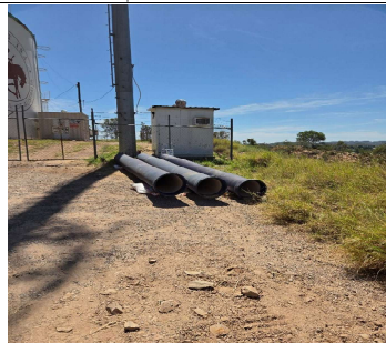
Pipe Storage at Reservoir 2 Alignment
