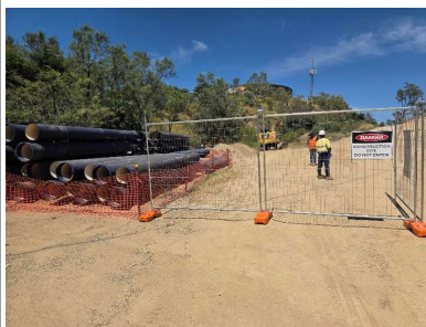
Pipe Storage Compound off Sutton St
