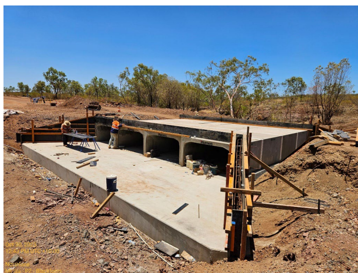
Figure 1 – Culvert Construction on Gunpowder Road
