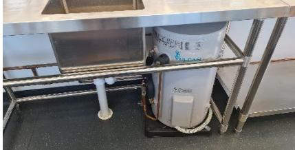
A stainless steel sink with a hot water system underneath, including a large white tank and piping. |
