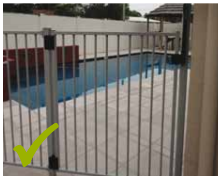
This gate is self-closing and in good condition.
