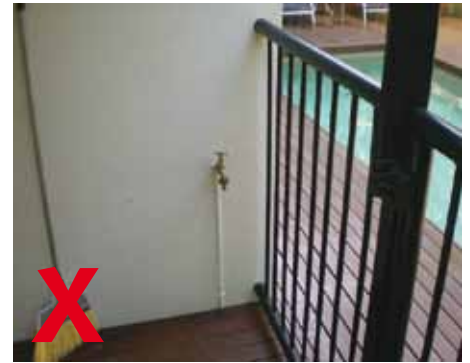
A tap fitting is a climbable object and must be shielded or removed.
