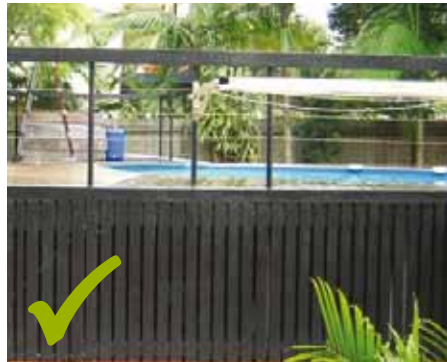
This deck bracing has been covered up with vertical palings.
