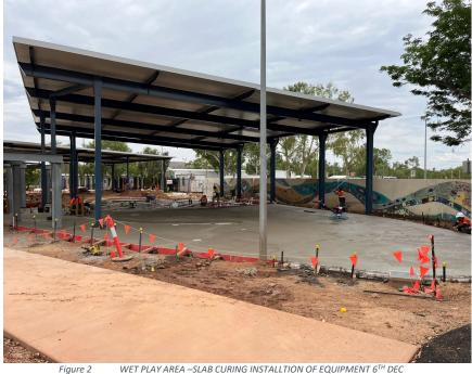
Figure 2 WET PLAY AREA –SLAB CURING INSTALLTION OF EQUIPMENT 61" DEC
