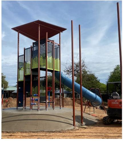
Figure 4 TOWER 1 COPPER CITY – READY FOR SOFT FALL AND ROPE BRIDGE CONNECTIONS ROPE BRIDGE DELAYED 20 TH DEC
