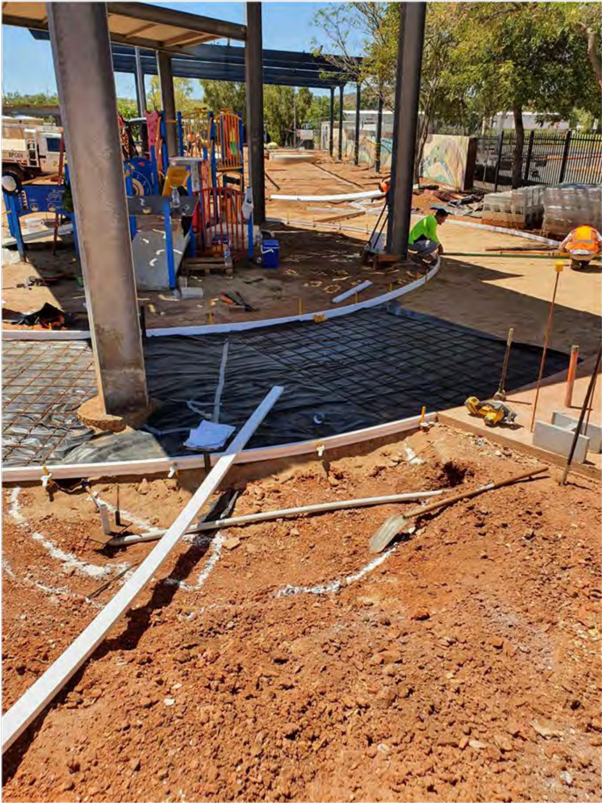
RIGHT PICTURE: STEEL WORKS TO CIRCULAR FOOTPATH
