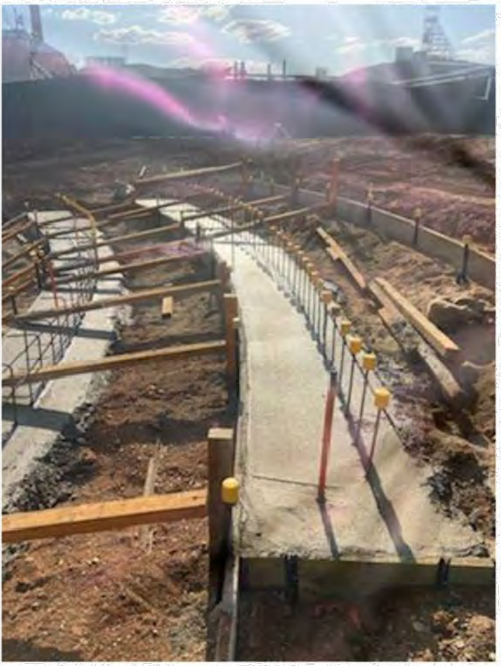
RIGHT PICTURE: Concrete pour for the second tier of the in mound seating
