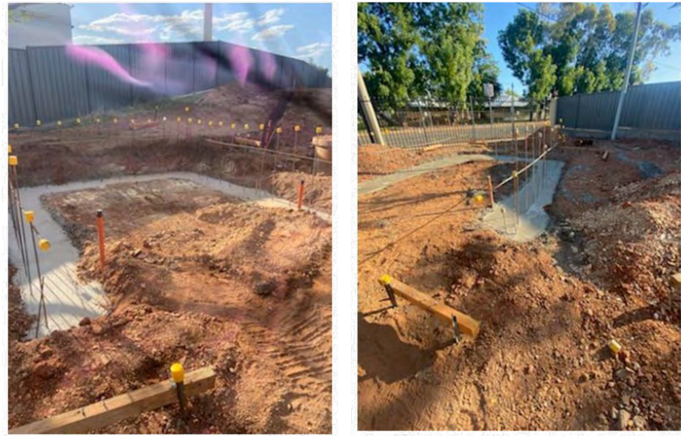
LEFT & RIGHT PICTURE: Foundations for picnic and BBQ area retaining wall
