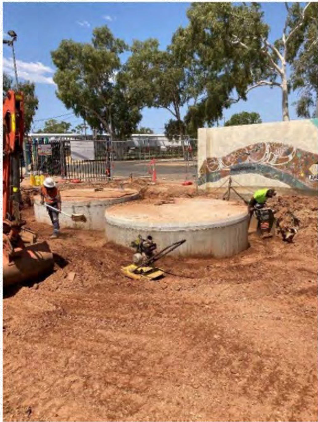
LEFT PICTURE: Backfilling 3m deep balance tank. Preparing for the wet play hydraulics
