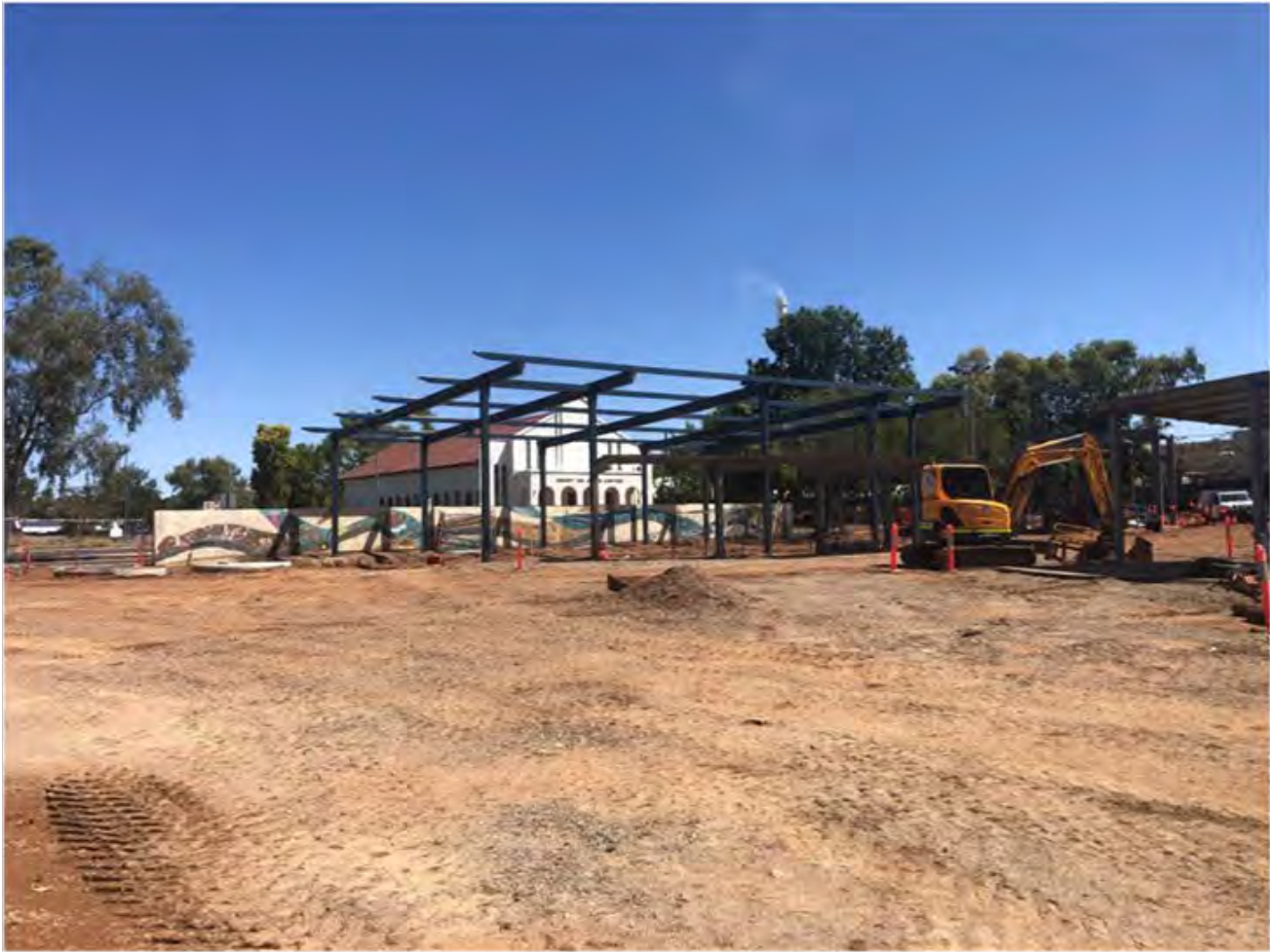
RIGHT PICTURE: WET PLAY SHADE STRUCTURE – STEEL WORK COMPLETE
