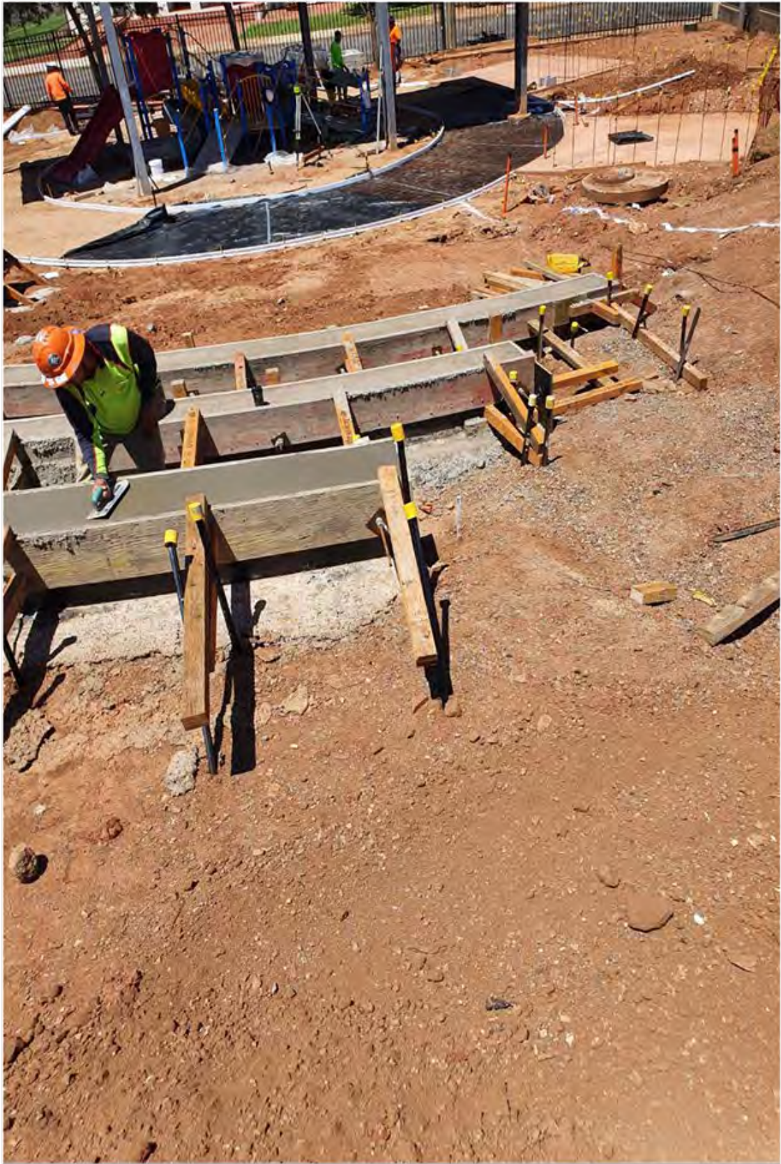
LEFT PICTURE: CONCRETE FINISHING WORKS TO IN MOUND SEATING
