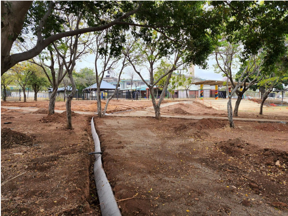
Completed stage removal, earthworks to regrade existing retaining wall and drainage, pre fabricated steel for seats and interpretive signage. Subbase material for footpaths and spine. Hold down bolts and civil works complete for Amphitheatre shade structure parklands, drainage
