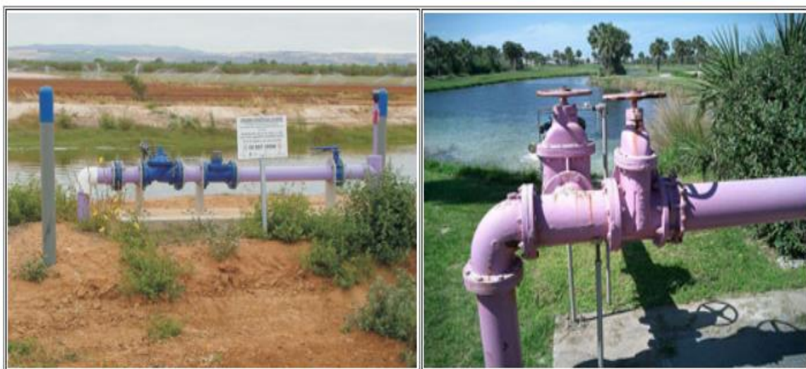
Examples of the purple/lilac plumbing to denote use of recycled water.
